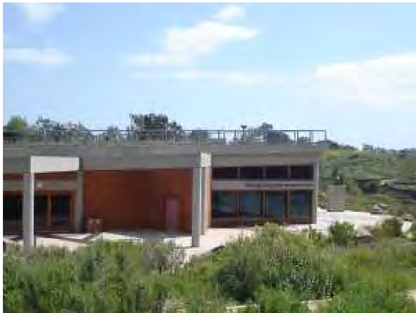
Figure 8 – UNBNR Muth Interpretive Center (not visible from adjacent land development, by design)
