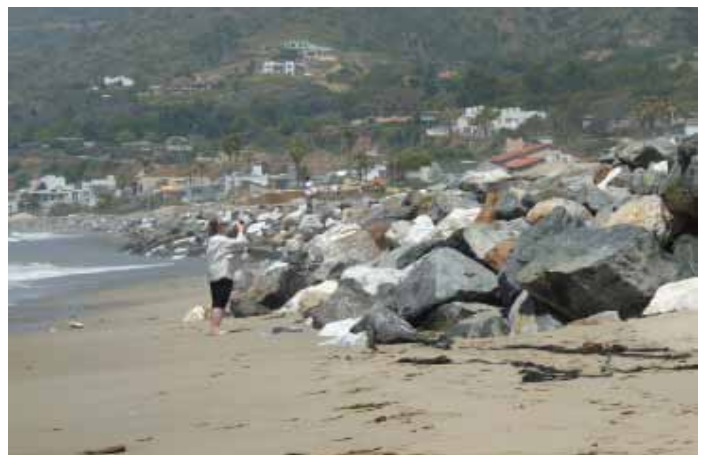
Along Broad Beach, emergency rock revetment was built to protect homes built too close to the shoreline. Now, sea level rise due to climate change will bring exacerbated flooding to parts of the coast such as Broad Beach (Image credit: Phyllis Grifman)
