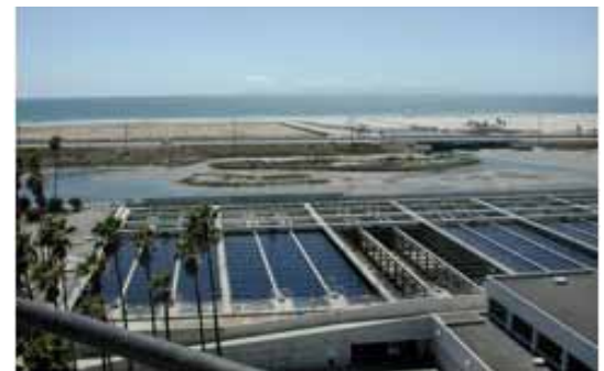
The Southern California region has one of the largest wastewater effluent systems in the country, contributing more than one billion gallons of treated wastewater to the ocean daily, making treated wastewater the largest source of fresh water inputs to marine waters. (Photo credit: Phyllis Grifman)
