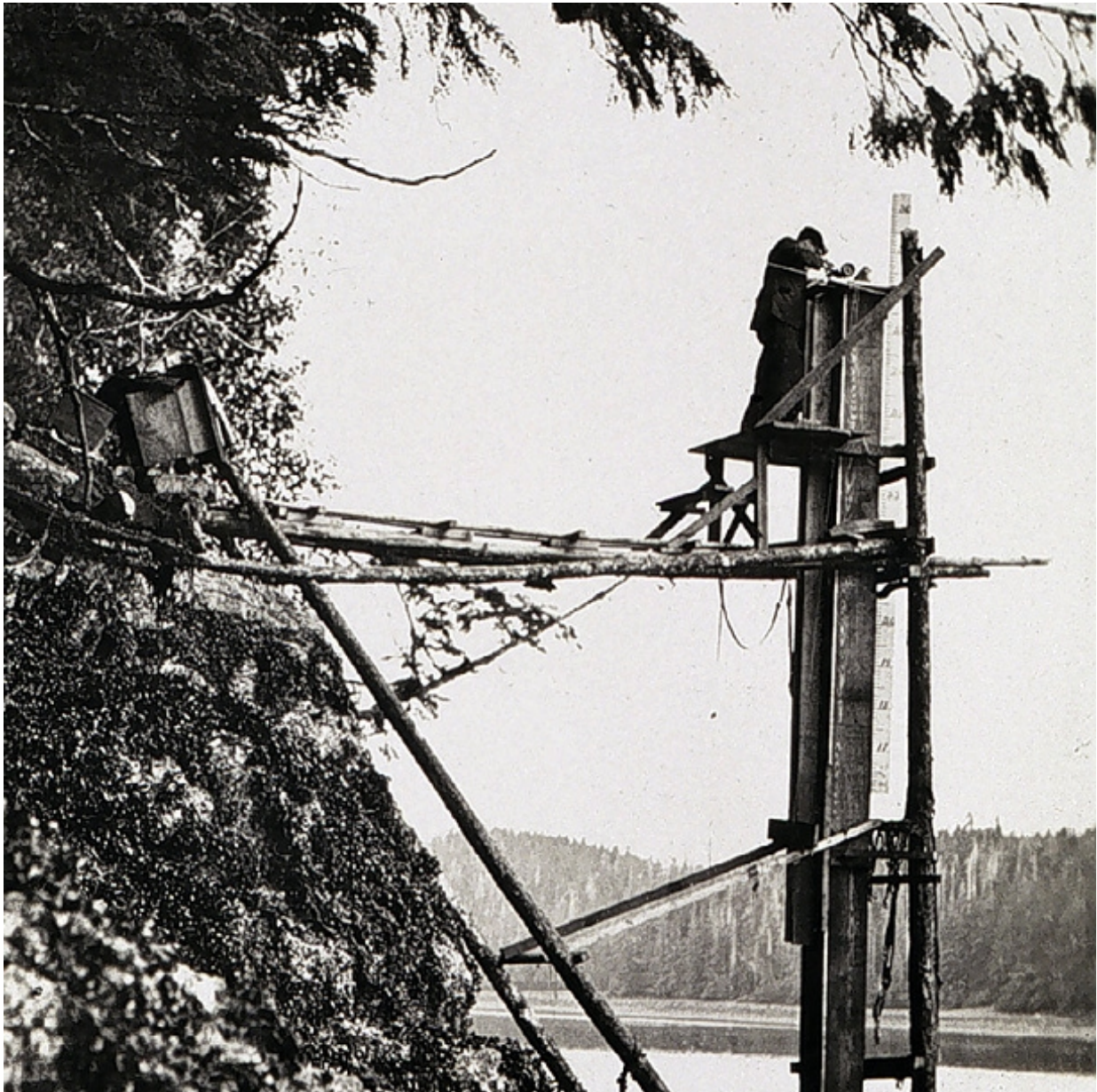
Checking the automatic tide gauge at Port Protection, Prince of Wales Island, Alaska, 1915. Photo from NOAA Photo Library.
