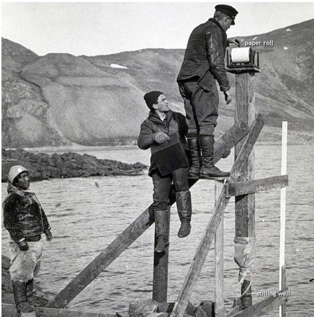
A Coast and Geodetic Survey officer (B. H. Rigg) checking a tide gauge on western Greenland as part of the MacMillan Arctic Expedition in 1926. Original photo from NOAA Photo Library.
