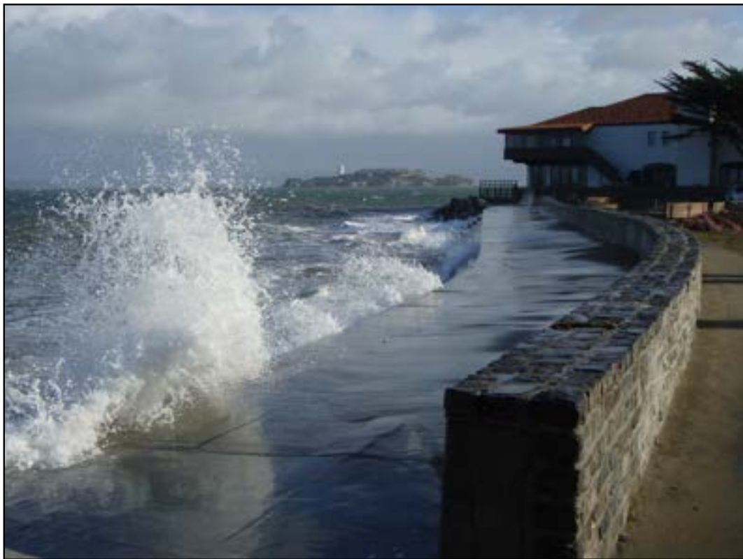
High water over the St. Francis Yacht Club San Francisco, CA, during a king tide on Jan. 21, 2012. Photo credit: Matt Richardson.
