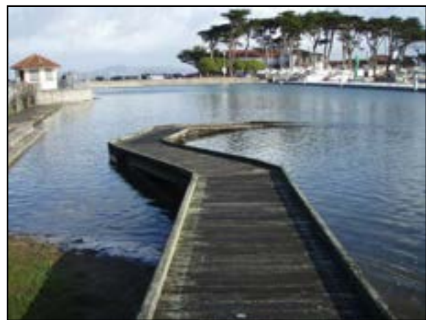
Pedestrian/Disabled ramp in the Marina District, San Francisco, CA, during a king tide on Jan. 21, 2012. Photo credit: Matt Richardson
