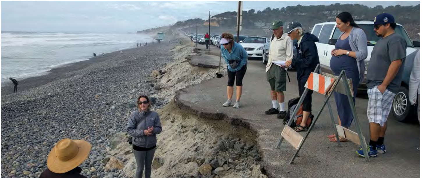
Dr. Sarah Giddings (on the sand) explains how high tide combined with storms can cause damage to infrastructure. Credit: Astrid Hsu
