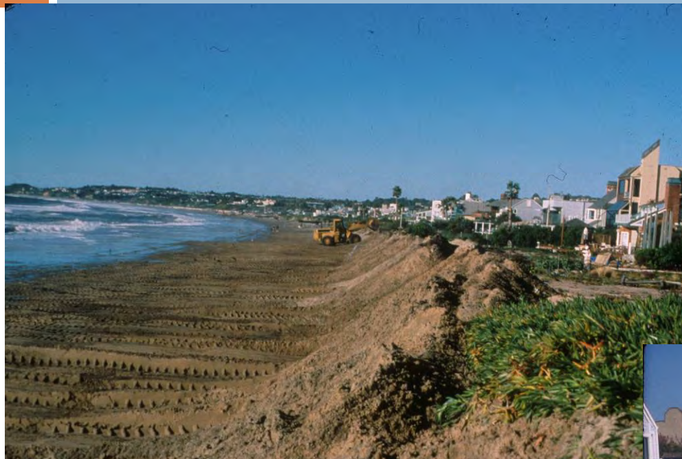
Berm Building/ Beach Scraping
