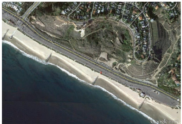
Google Earth image of Will Rogers State Beach with effective groin beach stabilization.
