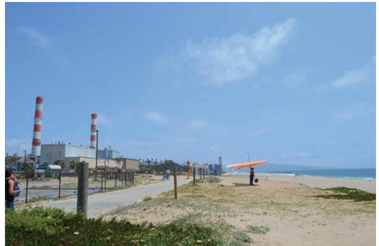
A sand dune protects a L.A. power generation plant while residents enjoy coastal recreation. (Photo credit: Marika Schulhof)
