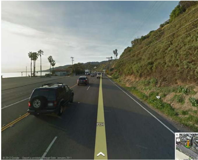
FIGURE 4: THE PACIFIC COAST HIGHWAY IN PACIFIC PALISADES, SHOWING ITS LOCATION WEDGED BETWEEN THE SHORELINE AND THE HILLSIDE. MOST PORTIONS, LIKE THIS ONE, HAVE PARKING LOTS ALONG THE BEACH FOR PUBLIC ACCESS TO THE SHORE (SOURCE: GOOGLE MAPS)
