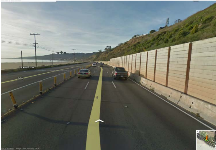
FIGURE 5: PACIFIC COAST HIGHWAY LIES BETWEEN AN ERODING HILLSIDE (RETAINING WALL SHOWN ON THE RIGHT IN THE PHOTO) AND THE BEACH AT THE SOUTHERN PORTION OF THE CITY LIMITS ALONG PACIFIC PALISADES' STRETCH OF COASTLINE (SOURCE: GOOGLE MAPS).
