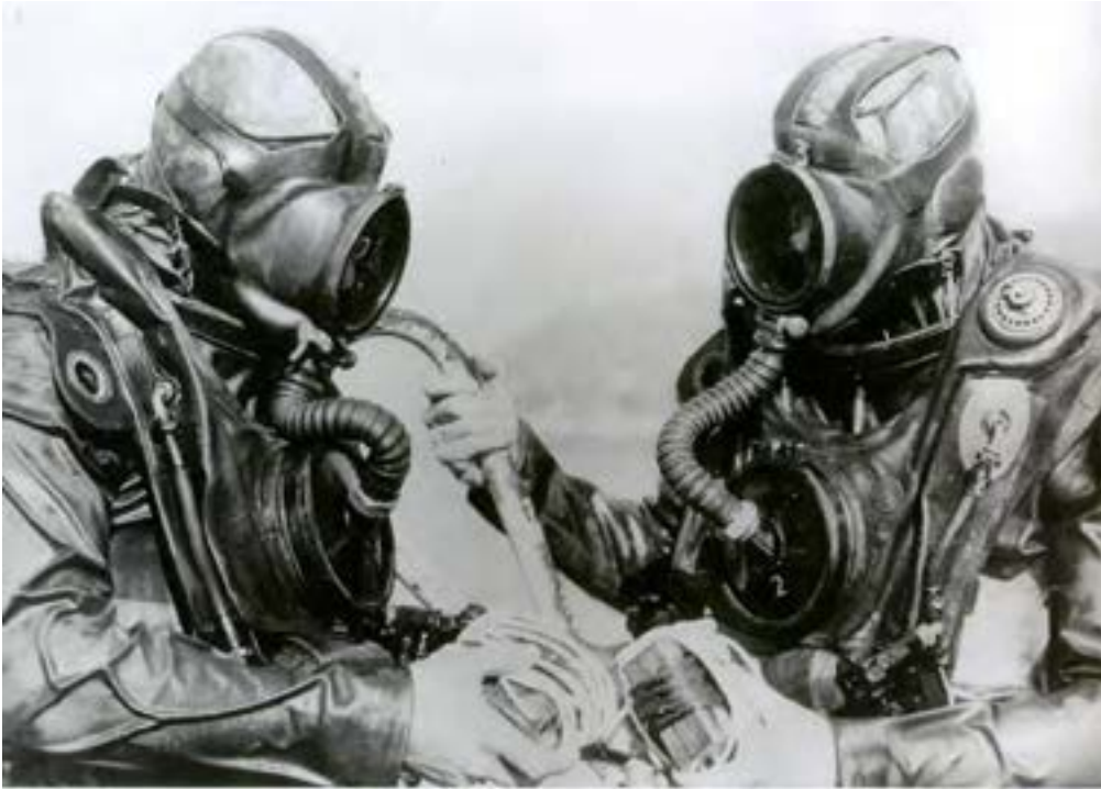
Fig. 5.19 Military diver wearing oxygen rebreathing sets.
